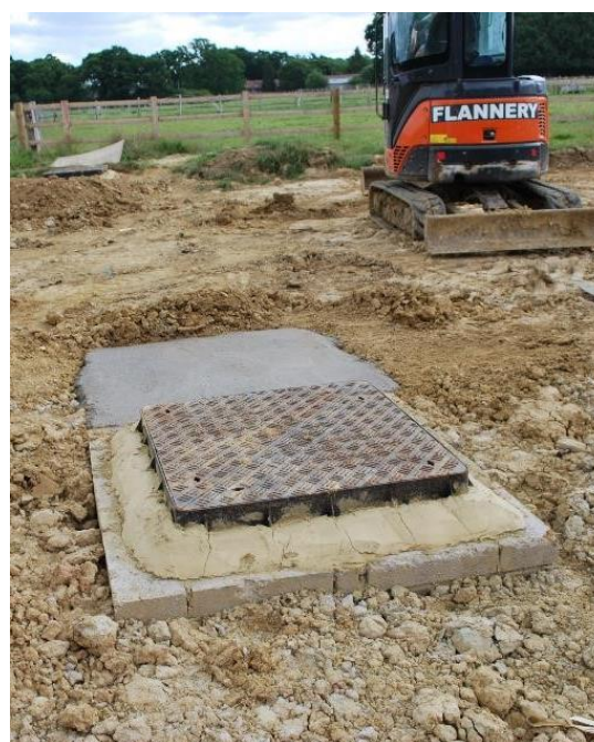
Figure 1.13 A: A typical jointing pit under construction. B. typical link box cover once backfilled (image courtesy of RWE Renewables)
